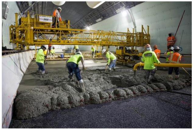
Crew workers laying the final section of concrete (credit: portofmiamitunnel.com)
