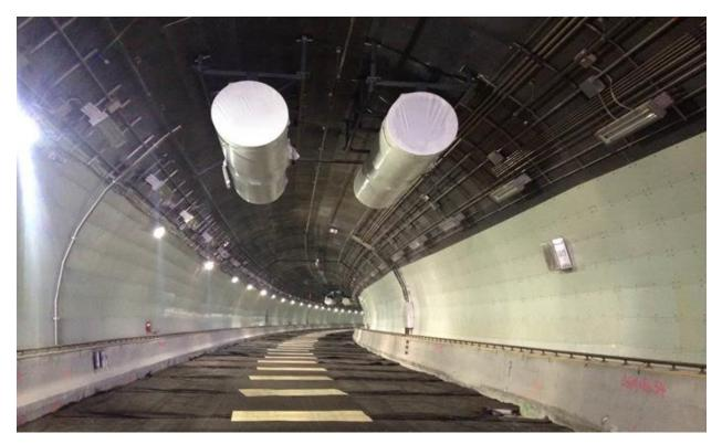
Jet fans in Miami Tunnel during construction (credit: portofmiamitunnel.com)
